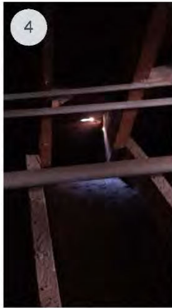
Picture take from attic interior showing hole in slate roof.
