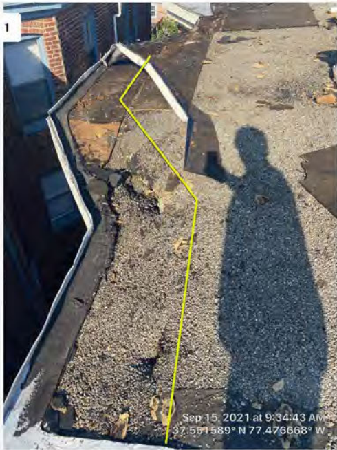
Picture showing area of rotten wood in built in gutter system.
