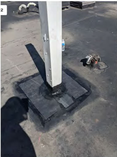
After picture of new EPDM target patch and flashing installed around deck post.
