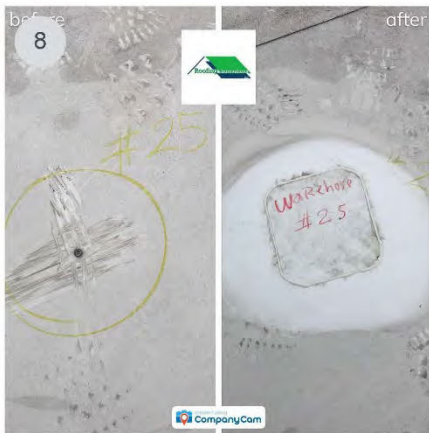
Before and after picture of TPO patch installed over puncture hole in membrane.
