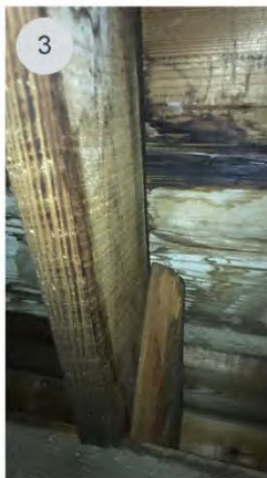
Picture showing small amount of water staining from attic.
