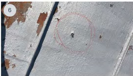
Picture showing nail hole in metal roof.
