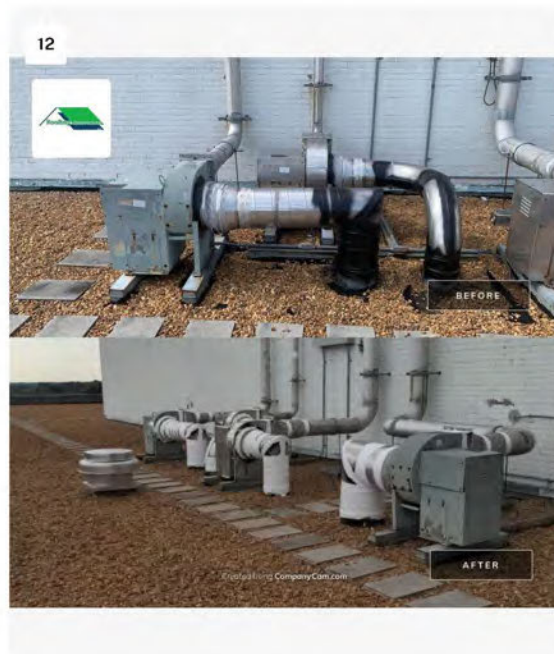
Before and after picture of seam sealer mastic flashing applied to seams on HVAC ducts.
