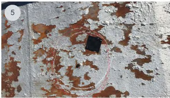
Picture showing nail hole in metal roof.
