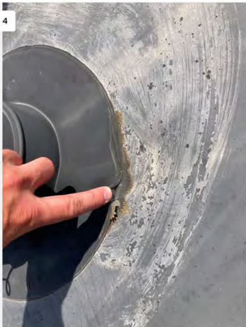
Picture showing open seam on EPDM pipe boot. Permanent repair: Remove and replace EPDM pipe boot.
