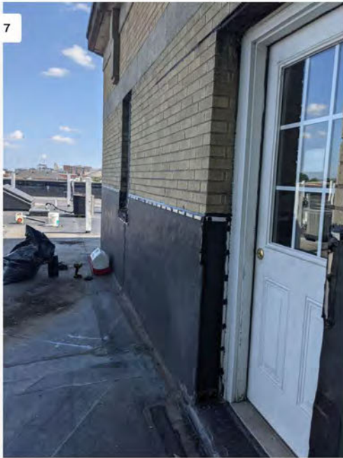
After picture of new sealant applied to termination bar on wall flashing.
