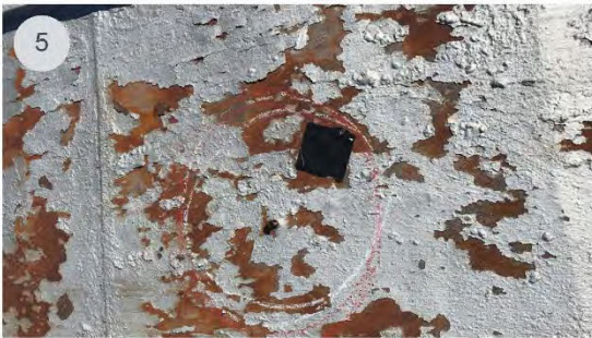
Picture showing nail hole in metal roof.
