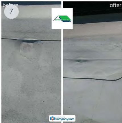
Before and after picture of TPO patch installed over open seam in membrane.
