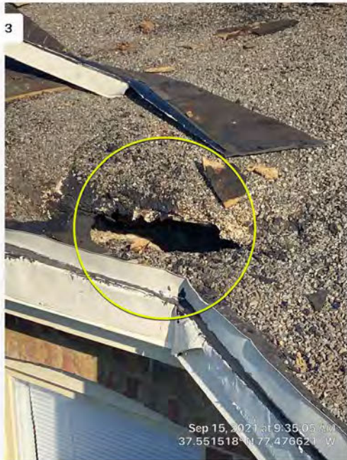
Picture showing hole in roof decking. Rotten decking and rafters throughout built in gutter.
