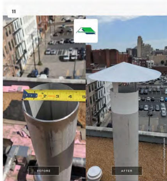
Before and after picture of HVAC duct caps installed.
