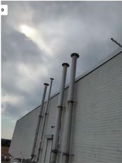
After picture of HVAC duct caps installed.
