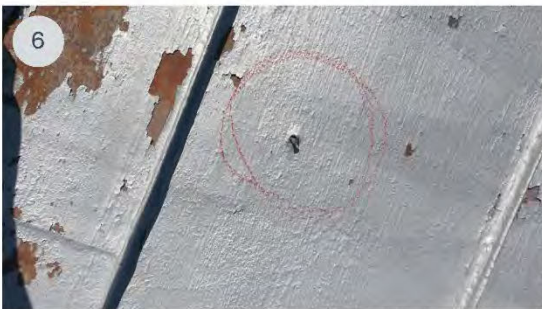
Picture showing nail hole in metal roof.
