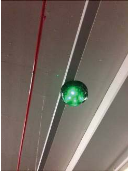
Sample Single Space Installation (Uni-Strut/Rail Installation):
