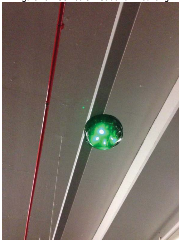
Figure 16: TUS-100 Uni-Strut/Rail mounting
