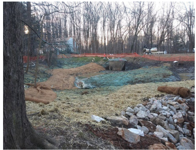
Monarch Lane, Post Construction
