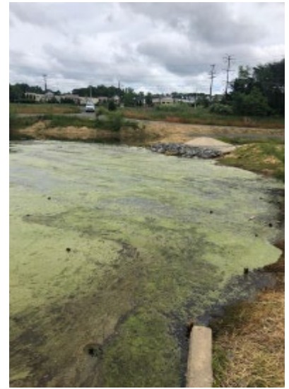
Fair Ridge Pond, Post Construction
