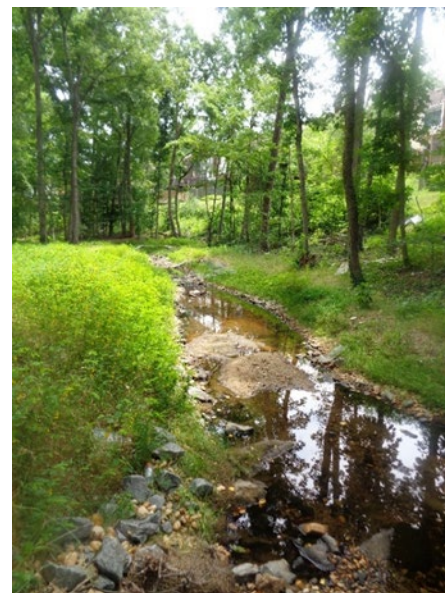
Occoquan Reach 5, post-construction
