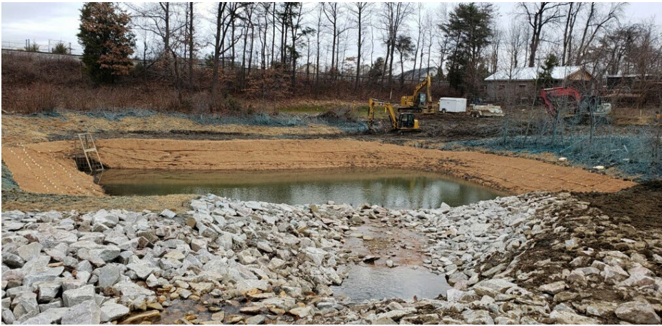
Vine Street. Post-Construction
