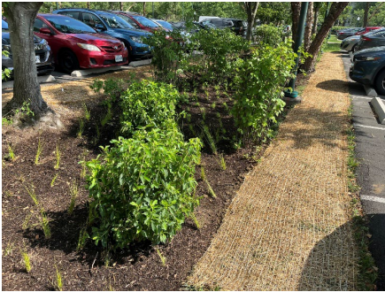
Side slope stabilization
