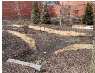
Border stone displacement
