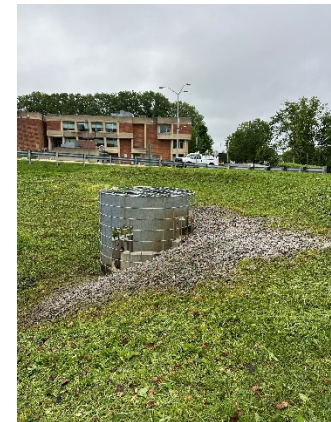
Control Structure Cleaning
