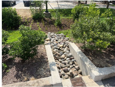
Inlet protection stone cleaned
