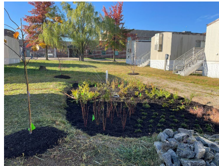
After new bio-retention construction
