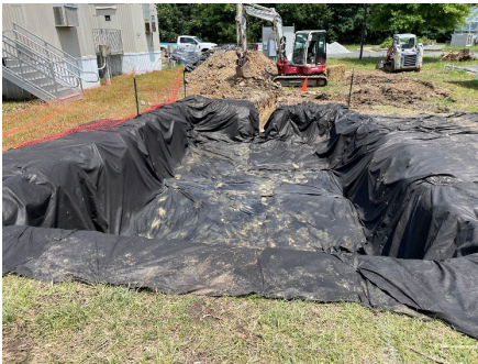
During new bio-retention construction
