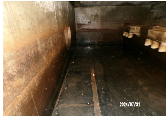
After sediment/debris removed from structure
