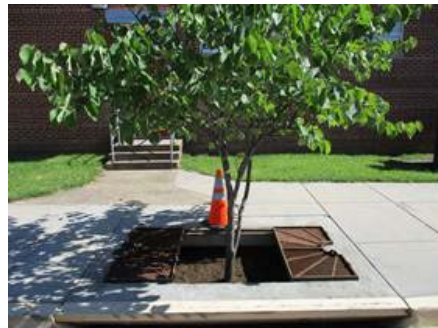
Single unit Filterra tree box filter
