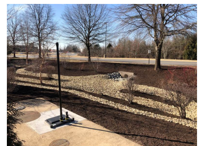
Facility stabilized with mulch/stone
