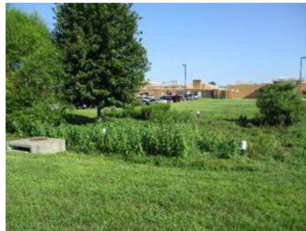
Bio-retention overall view
