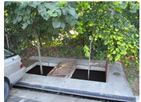
Dual unit Filterra tree box filter
