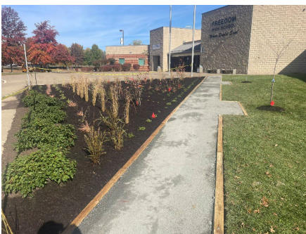
Crushed stone walkway at native garden
