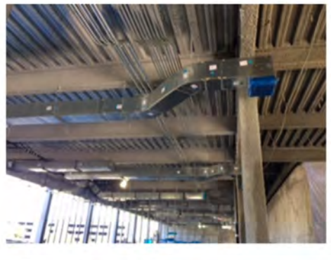
Virginia Tech – New Classroom Bldg Field Installation
