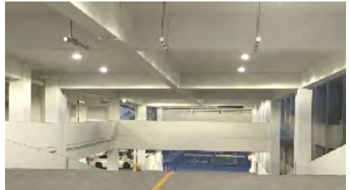
Ultrasonic directional sensors monitor vehicle entry exit at garage/level entry exit.
