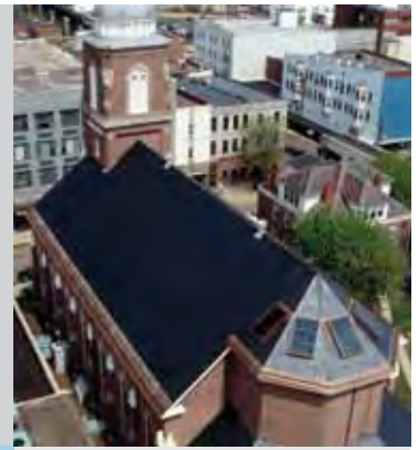
Above: Our team replaced wood decking, slate shingles, and copper flashing on this 19th century Gothic structure.
