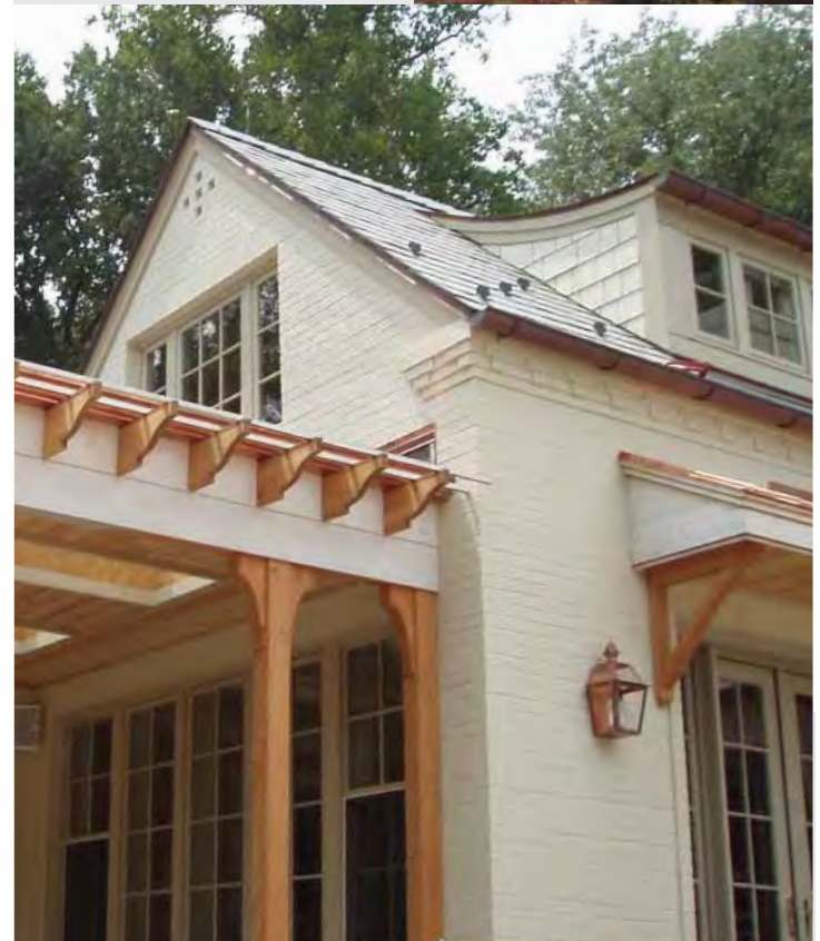
Above: New residential Vermont slate installation with custom-fabricated half-round copper gutters and standing seam copper dormer roofs.
